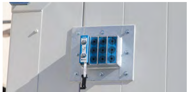
Cable box (fire bulkhead) for the passage of cables through the wall of the fire-rated store, while maintaining the fire resistance of the component
